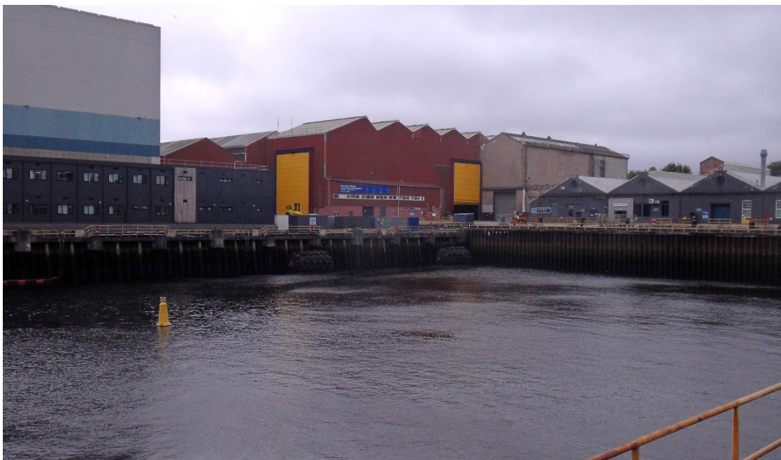
Photo 5.2: View facing south-east across the Fitting-out Basin (MM054) towards MM007 (not directly visible behind later extensions).
