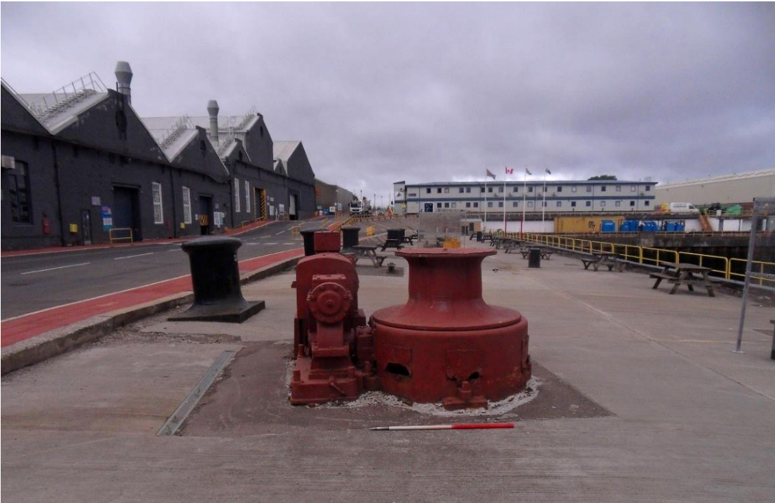
Photo 5.8: View facing west at the south-eastern end of the Fitting-out Basin (MM054) showing the winch (MM096) in the foreground along with several mooring posts in the background (MM095).
